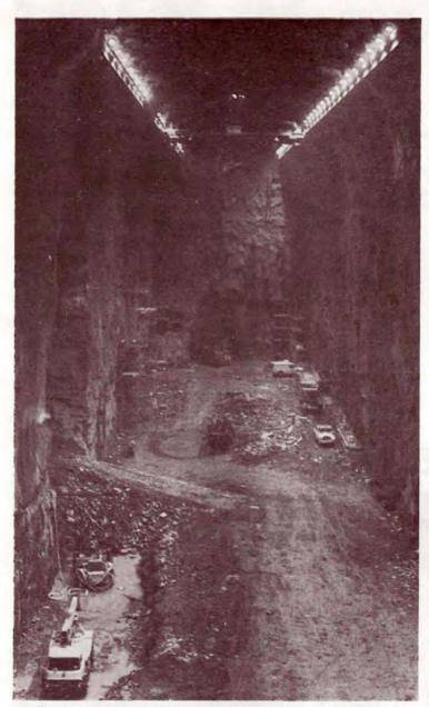
"The underground chamber housing the main plant will be one of the largest excavated caverns engineered in the world—twice as long and half as wide as a soccer pitch, and higher than a 16-storey building." These are the words of a CEGB booklet on Dinorwic. Our picture shows the still-unfinished reality, with lorries and vans looking like toys. More than two million tons of slate will have been excavated when Dinorwic is complete.
